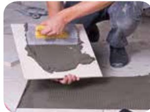
Double sided adhesive bonding should be used on ceramic applications over 20x20 cm (both to the surface and back side of ceramic), and the tooth size should be increased.
