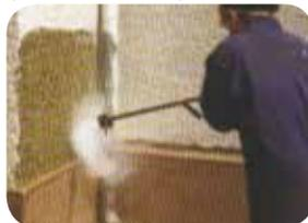
**SAND BLASTING:** It is the process carried out as a result of spraying of the special materials called as sand, looking like sand but actually different than sand known by us and manufactured specifically for this work and having types such as silica, basalt, grit and different places of use by means of compressed air onto surfaces to be painted.
