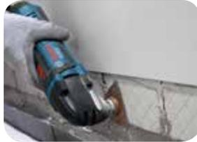
**GRINDING:** It is the process of removal of the materials such as loose paint, paste and so on from the surface and removal of the burrs and threads on the surface carried out by using various grinding motors and grinding tips appropriate for the surface type.
