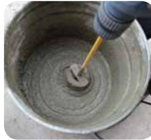
In order to obtain maximum performance from the products, it is necessary to comply with the water mixing ratios specified in the application instructions. If more water is added to the mixture, it may cause slipping after the bonding process and full efficiency cannot be obtained from the product. It is also recommended to mix the mortar with the mixer to obtain a homogeneous mortar mixture.
