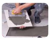
Double sided adhsive bonding should be used on ceramic applications over 20x20 cm (both to the surface and back side of ceramic), and the tooth size should be increased.
