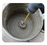
In order to obtain maximum performance from the products, it is necessary to comply with the water mixing ratios specified in the application instructions. If more water is added to the mixture, it may cause slipping after the bonding process and full efficiency cannot be obtained from the product. It is also recommended to mix the mortar with the mixer to obtain a homogeneous mortar mixture.
